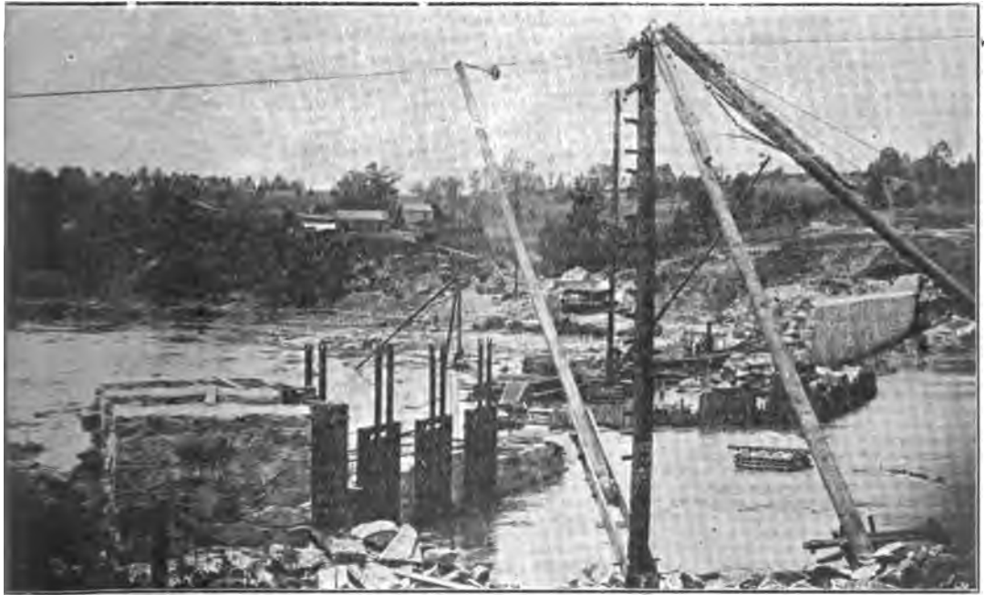
CONSTRUCTING A POWER DAM.
